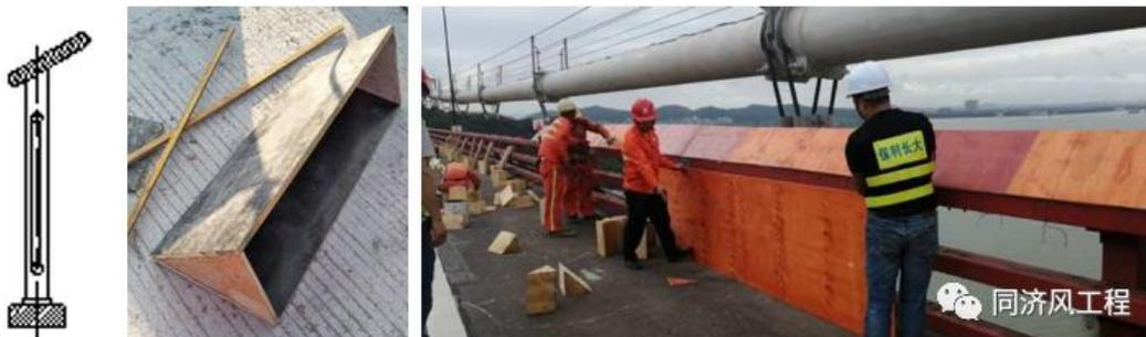
Fig.7 Experimental installation of spoilers (40 cm long, 45 degree inclination; continuous installation within 120 m on the upstream side and 70 m on the downstream side)
