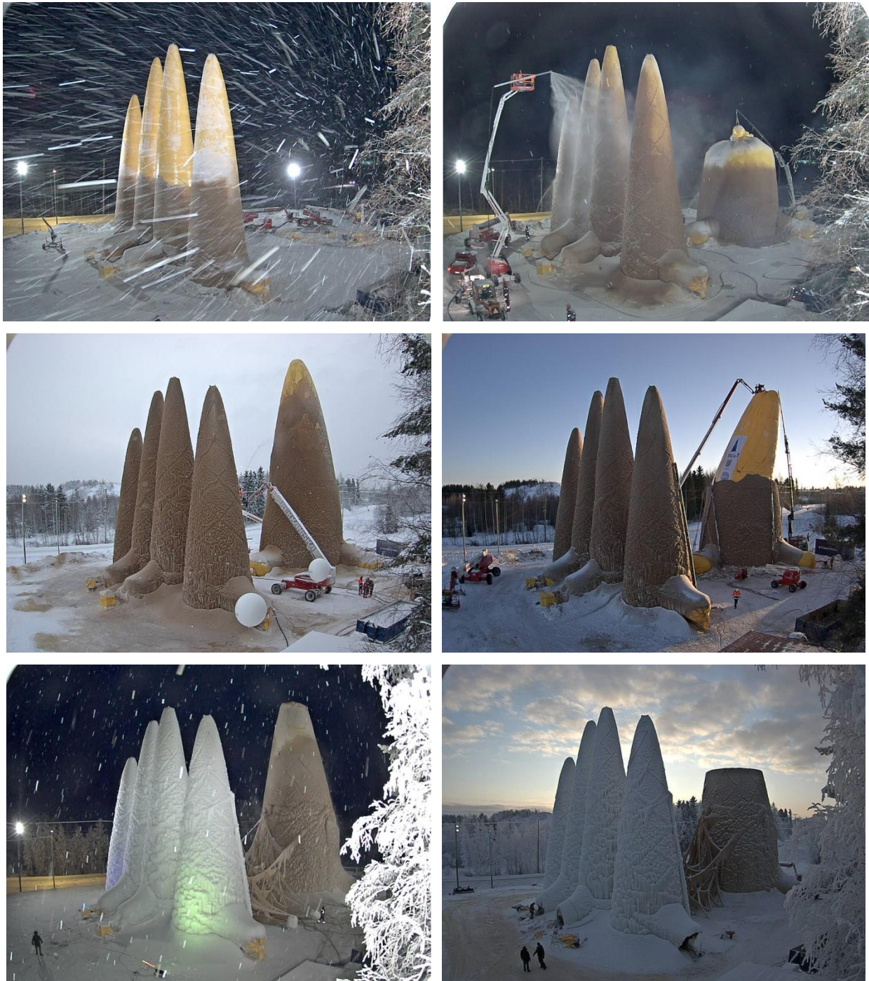
Fig. 6 Construction of the Sagrada Familia in ice – intermediary stages
