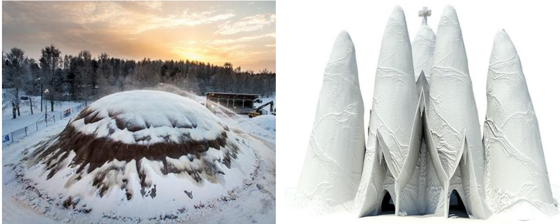
Fig. 1 Reinforced ice structures by Pronk et al. Left: picture of 30 m span dome, 2014. Right: Rendering of Sagrada Familia in ice, 2015.
