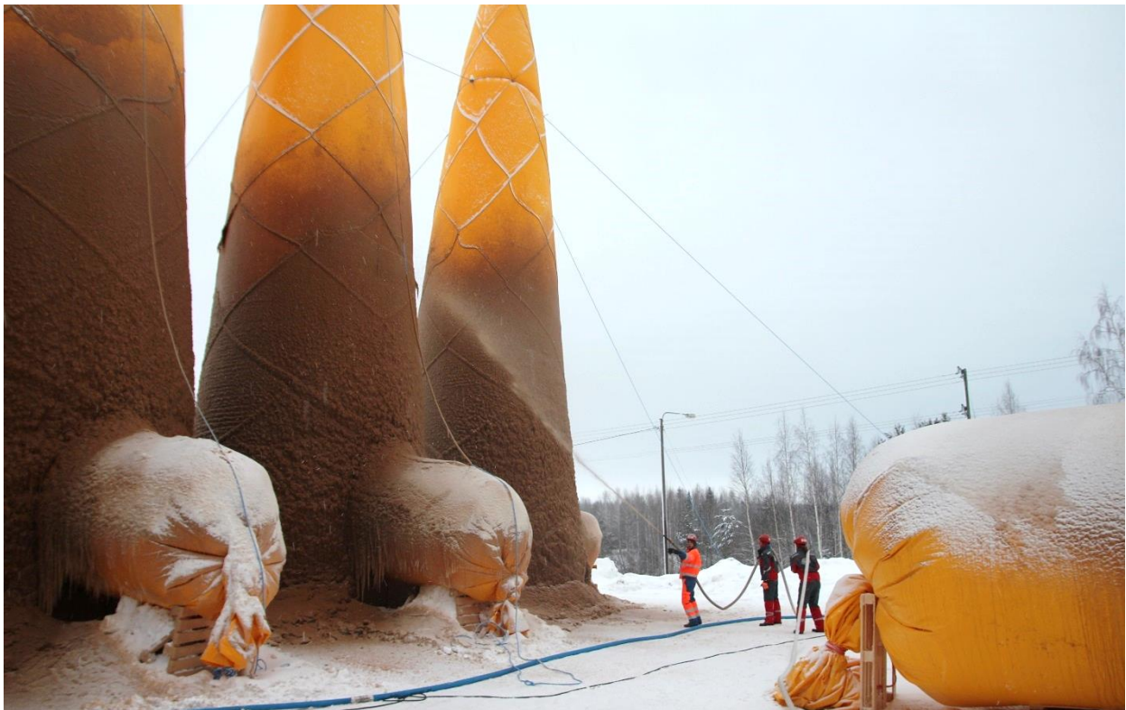
Fig. 4 Spraying of Pykrete onto inflated formwork of entrance towers
