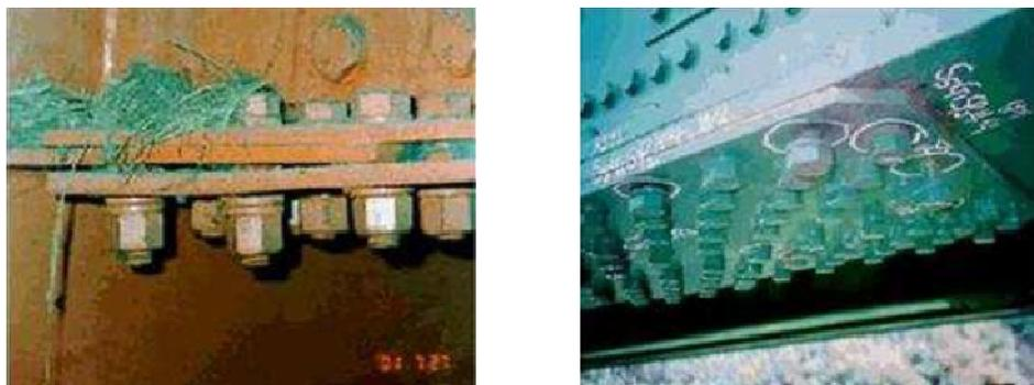
Fig. 2 Examples of completely loosened bolts
