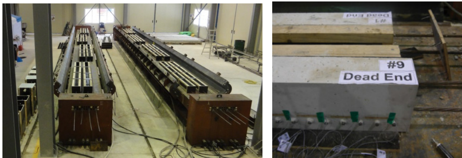
Fig. 1 Fabrication of pretensioned prestressed concrete beams
