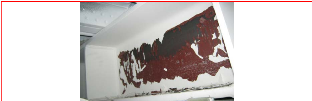
Fig. 10 Active link beam from Club Tower, Christchurch which has undergone
