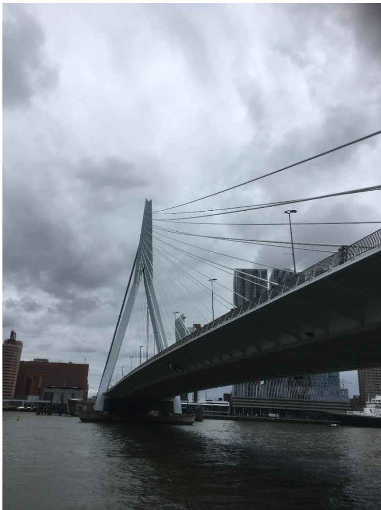
Fig. 2 Erasmusbrug, Rotterdam, Netherlands
