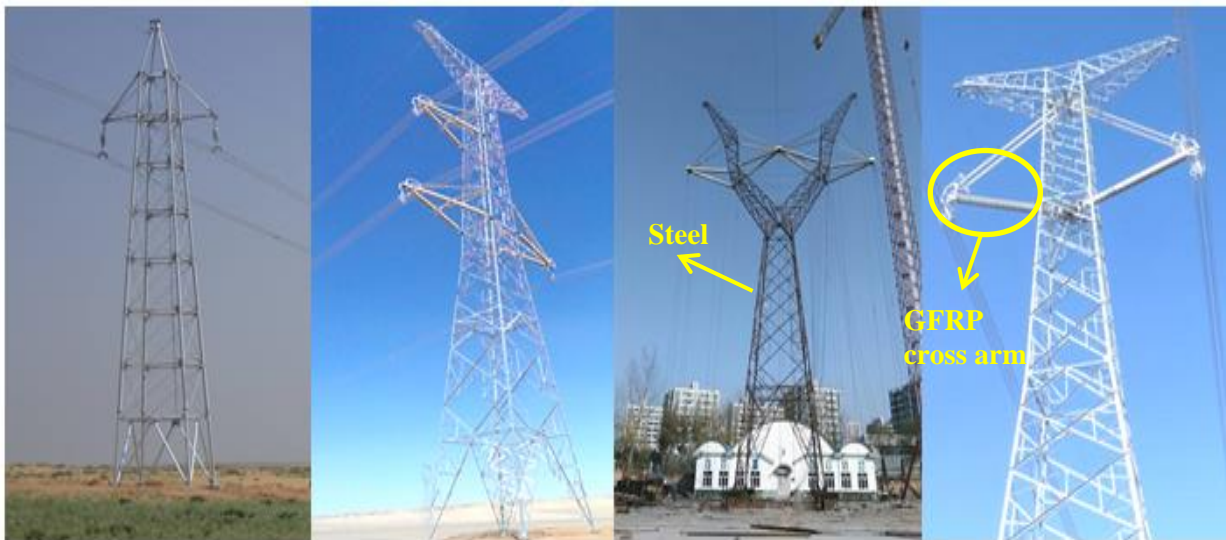
Fig. 2 GFRP-steel composite transmission towers
