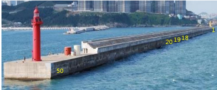
Fig. 4 The Oryuk-do breakwater of the port of Busan, Korea
