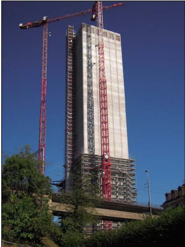
Fig. 9 Completed construction stage 4 in execution
