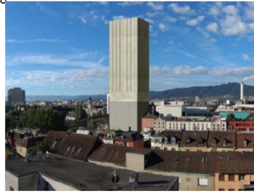
(b) after construction the new silo
