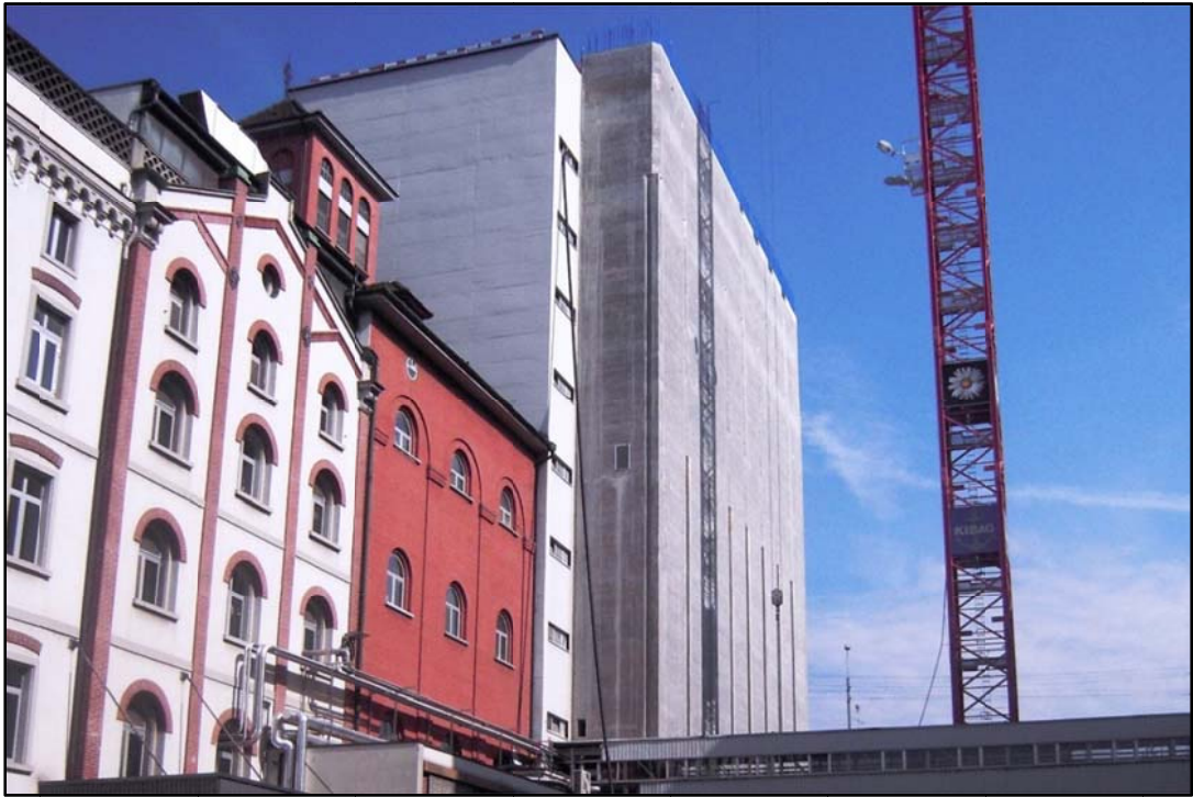
Fig. 8 Completed construction stage 1
