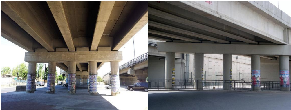
Fig. 2 Repaired/Retrofitted Bridges. (Photos: J.L. Seguel)
